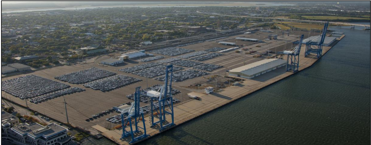
Figure 1-2: Aerial View of Columbus Street Terminal
