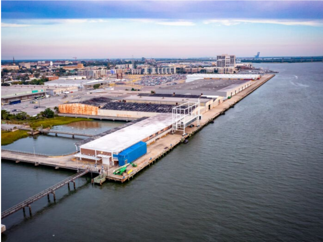
Figure 21: Union Pier Terminal (SC Ports Authority, 2024)
