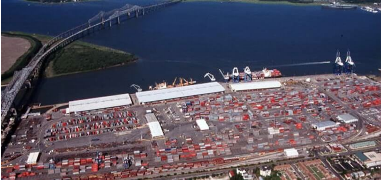
Figure 19: Columbus Street Terminal (Columbus Street Terminal – SSA Marine, n.d.)
