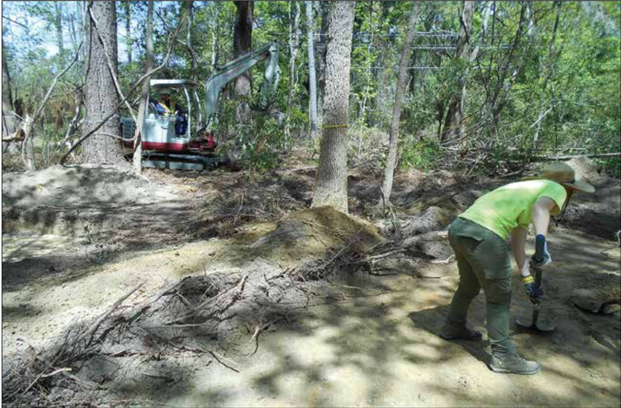
Figure 5.8 View of mechanical excavation in Locus 3.
