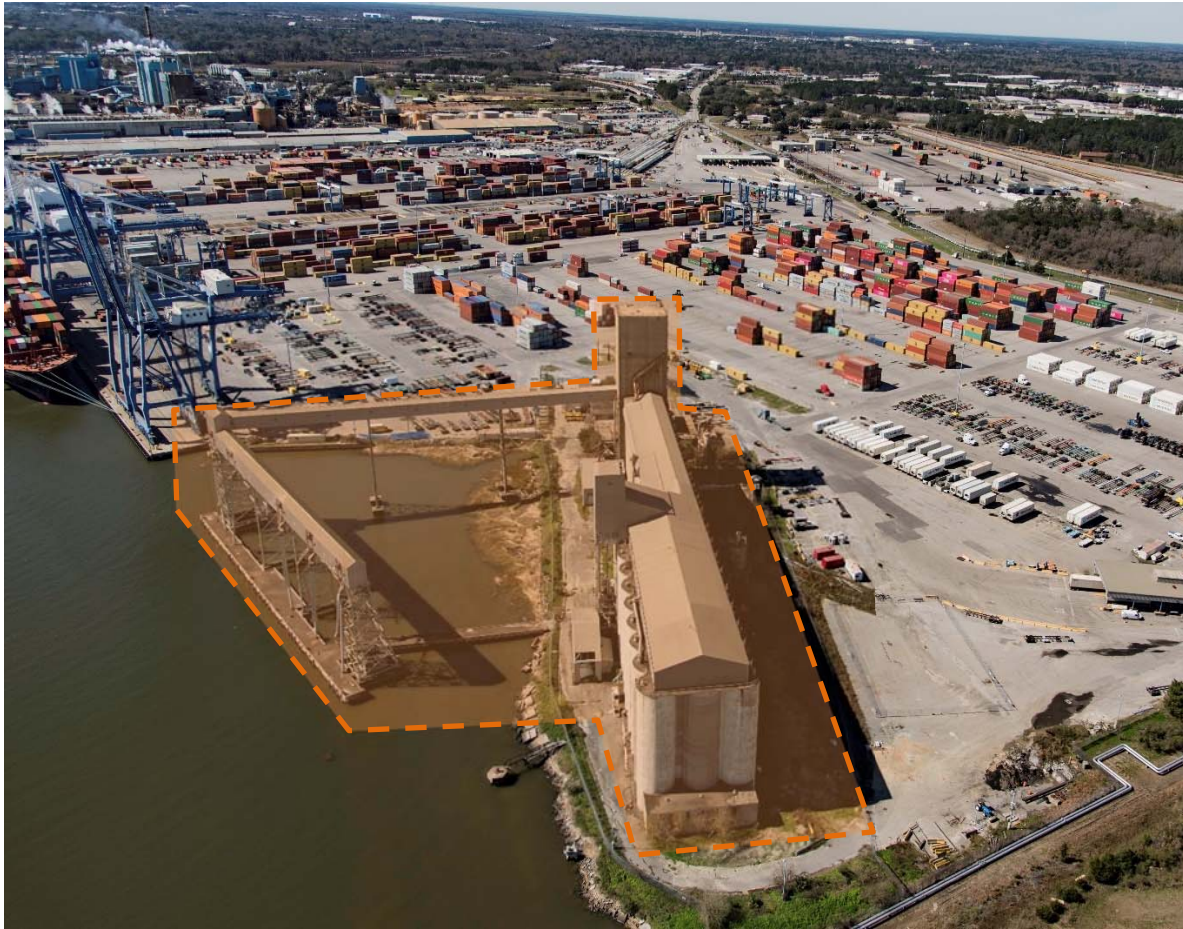
FIGURE 3: Area 10 Aerial Photograph
