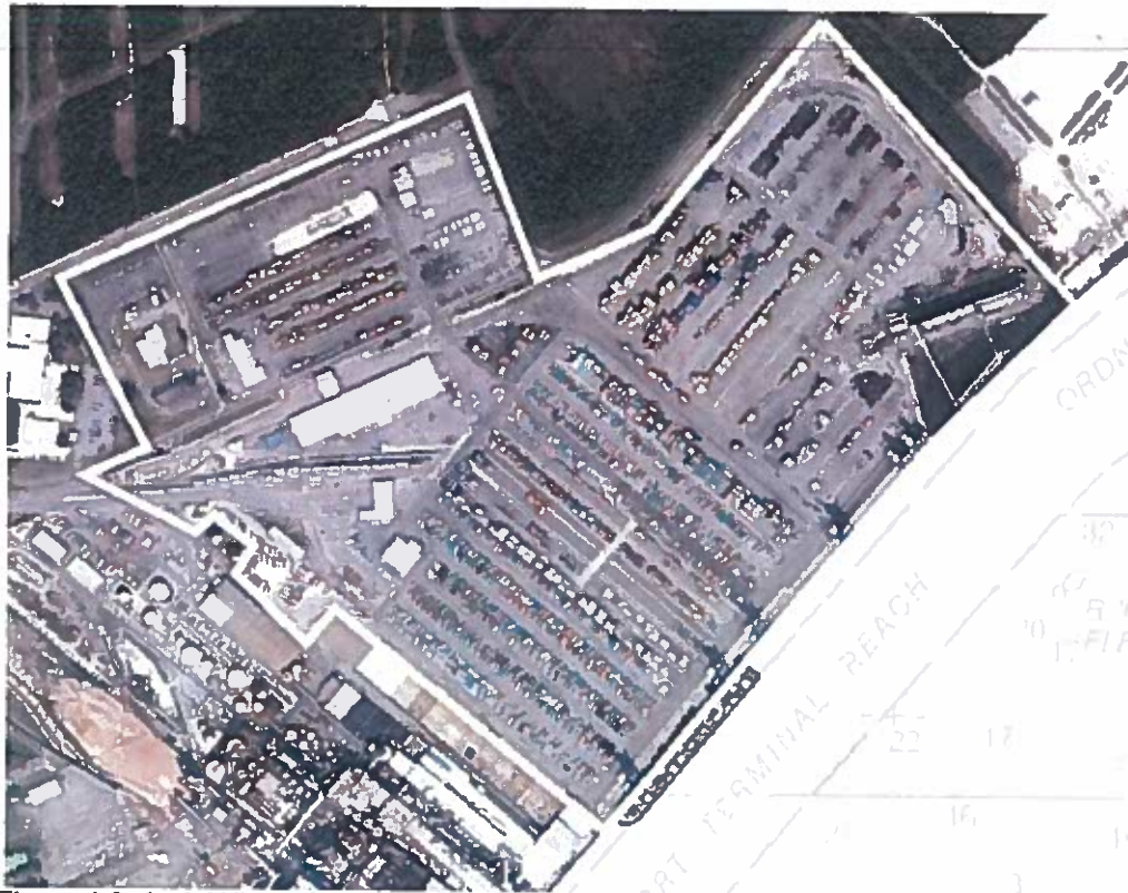
Figure 1-3: Aerial View of North Charleston Terminal
