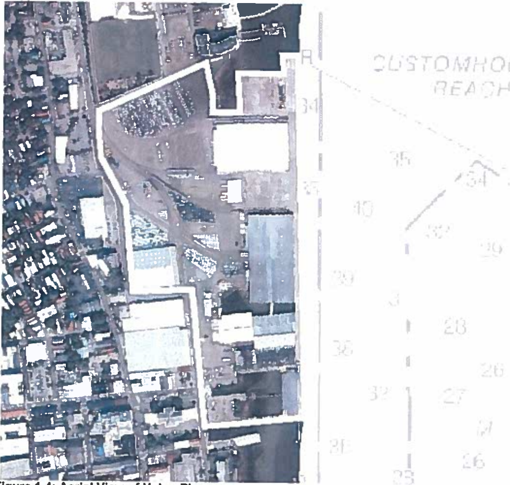
Figure 1-4: Aerial View of Union Pier
